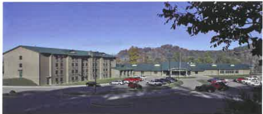
Above: Front facade of the Chief Logan State Park Lodge. The right conference center was completed in 2001 and the left guest suite addition was complete in 2006
